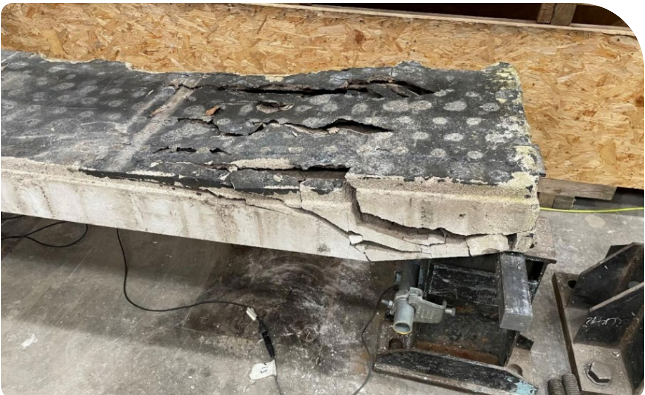
Figure 3: Shear failure of a RAAC plank during flexural test by Loughborough University and Lucideon Ltd as a part of the NHS-funded RAAC research programme undertaken in 2021-2023
