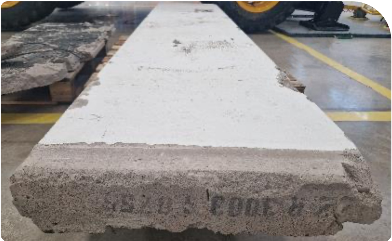
Figure 2: An upside-down roof plank sample, with soffit uppermost
