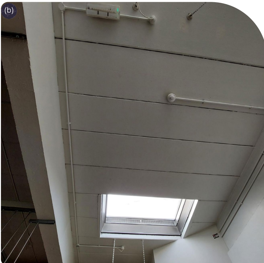
Figure 34: Hospital rooms where GPR trials were conducted. (a) Room #1, (b) room #2, (Source: MTC. With permission of Airedale General Hospital)
