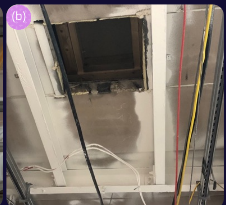
Figure 80: Parallel flange channels used for large span RAAC panel reinforcement in (a) large span hospital room, (b) around service cut out. (Source: MTC. With permission of Leighton Hospital) (c) Unistrut used to reinforce in space constrained areas (Source: MTC. With permission of Leighton Hospital)
