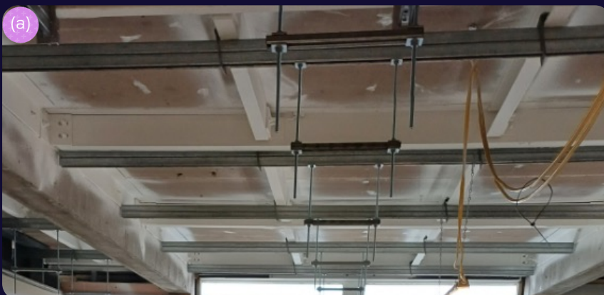
Figure 80: Parallel flange channels used for large span RAAC panel reinforcement in (a) large span hospital room, (b) around service cut out. (Source: MTC. With permission of Leighton Hospital) (c) Unistrut used to reinforce in space constrained areas (Source: MTC. With permission of Leighton Hospital)
