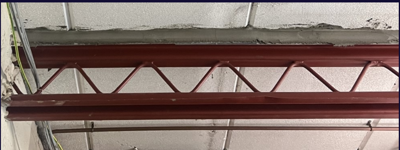
Figure 81: RAAC intermediate supports. (Image supplied by RAAC Consulting and Solutions ('RCS'))
